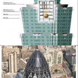
A Tuned Mass Damper (TMD), also called a "harmonic absorber", is a device mounted to a specific location in a structure, so as to reduce the amplitude of vibration to an acceptable level whenever a strong lateral force such as an earthquake or high winds hit. Some famous buildings with tuned mass damper include Shanghai Tower (Tallest building in China and world's tallest LEED Platinum certified building); Taipei 101, Taiwan
