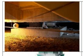
Museum of New Zealand Te Papa Tongarewa, Wellington by Ivan Mercep is protected from earthquakes by base isolators. The base isolators are made of a rubber-and-steel sandwich with a core of lead. The rubber gives flexibility, and the sheets of steel add strength. The lead core absorbs shock and turns some of an earthquake's energy into heat. In the 7.8-magnitude Kaikoura earthquake, the building 'slid' about 15 to 20 millimetres.
