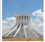
It was designed by Brazilian architect Oscar Niemeyer and calculated by Brazilian structural engineer Joaquim Cardozo. The cathedral is a hyperboloid structure constructed from 16 concrete columns, weighing 90 tons each.
